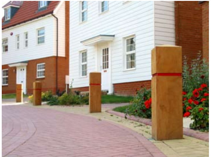
▲ EPPING with red reflective tape installed in Edenbridge, Kent
