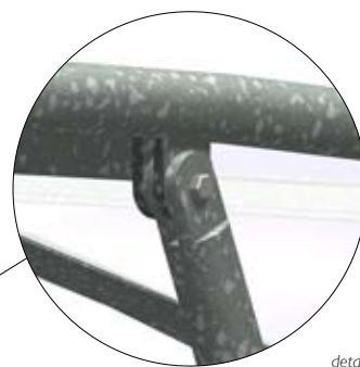
detail ROOF PURLIN SUPPORT BRACKET
