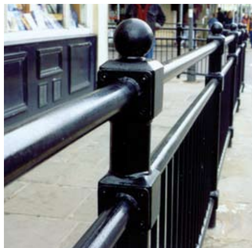
▲ HARRINGTON 3/4 GUARDRAIL installed in Greenwich, London
