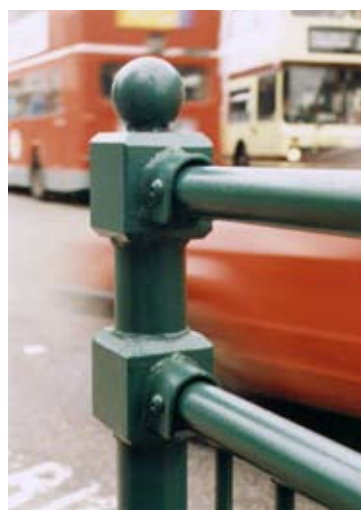
▲ HACKNEY 3/4 GUARDRAIL bracket detail supplied to LB Hackney
