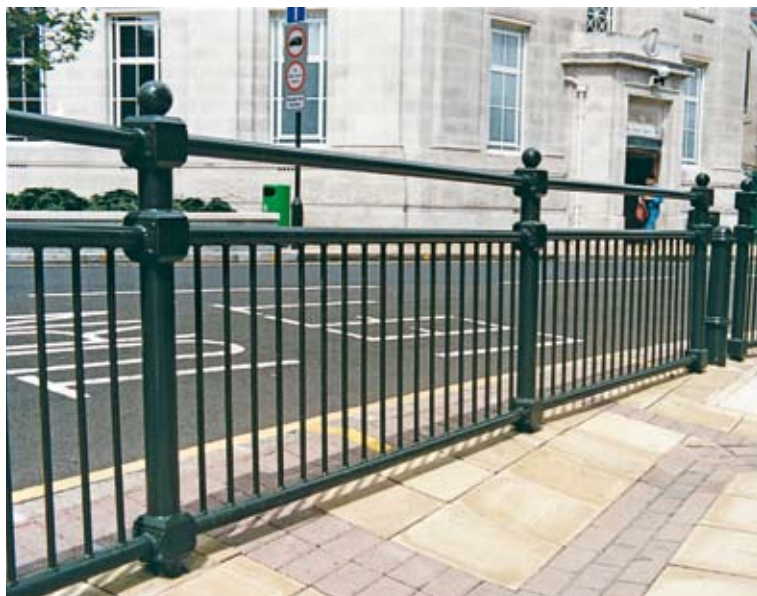
▲ HARRINGTON 3/4 GUARDRAIL as supplied to College Approach, Greenwich, London
