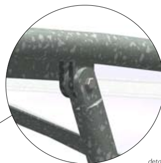
detail ROOF PURLIN SUPPORT BRACKET
